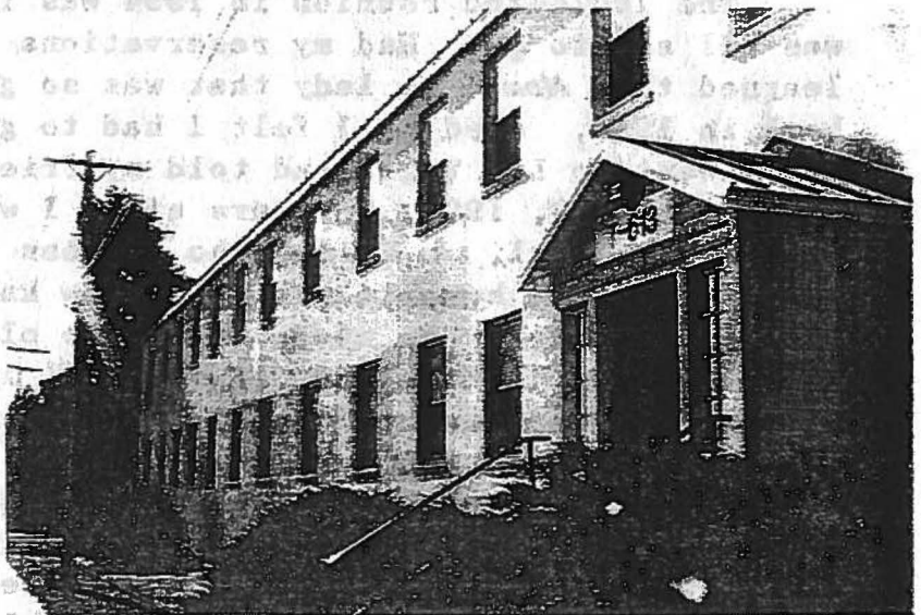
Left: The current gym is where Shimizu spent much time as an inpatient undergoing physical rehabilitation.
